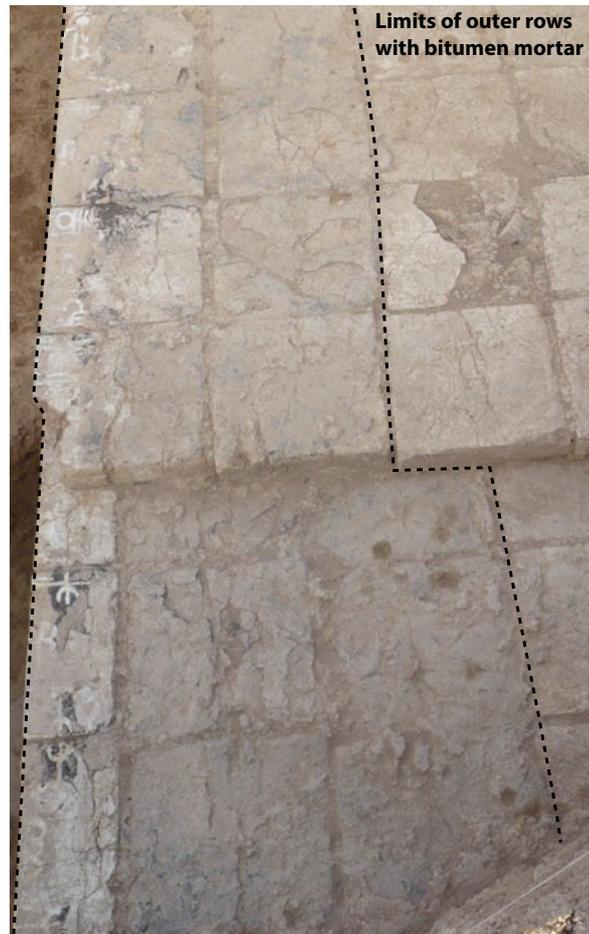
Fig. 18: Tr. 1, bitumen mortar on the outer rows of baked bricks of Block B
