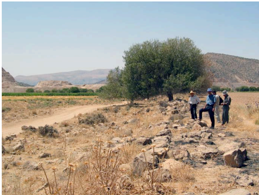
Fig. 18: A long rectilinear part of the “wall” (canal) on the left bank. It is made of two stone alignments together 2.20m in width.
