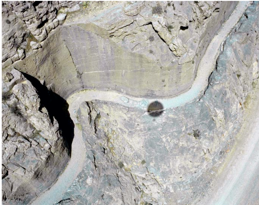
Fig. 14: The longest section (250m) of the rock-cut canal on the right bank of the Pulvar river.
