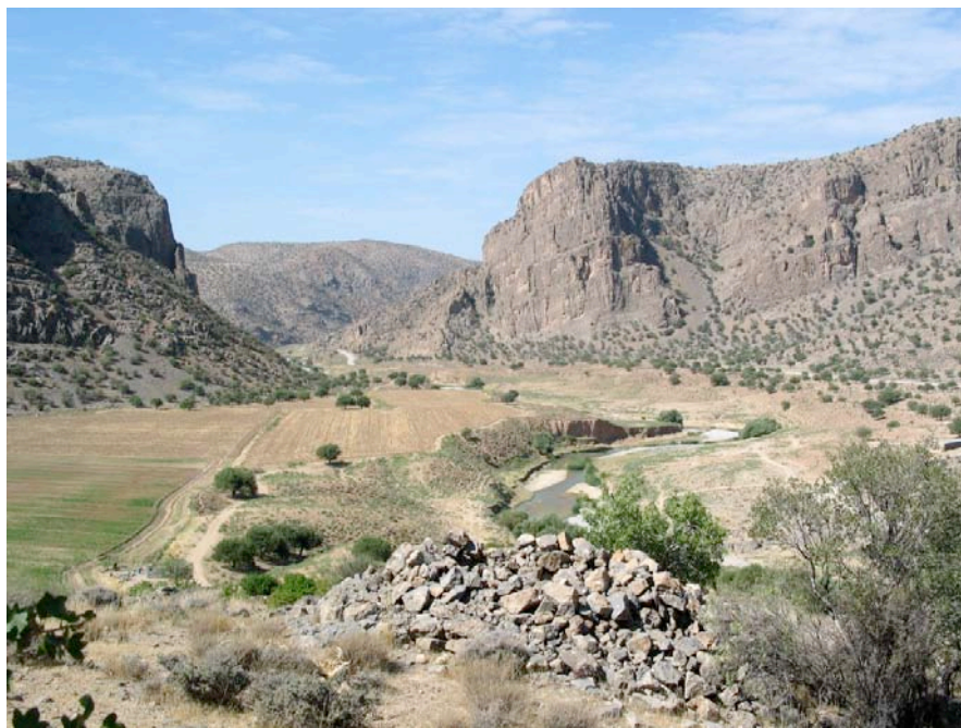
Fig. 1: General view of the narrowest part of Tang-i Bulaghi. On the right above, the longest section of the rock-cut passageway runs along the Pulvar river.
