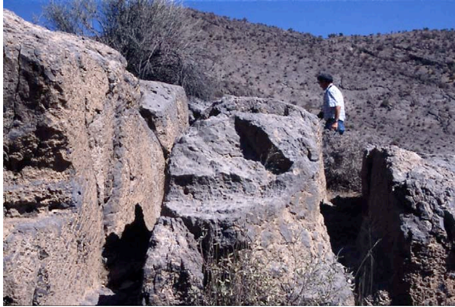
Fig. 15: An unfinished section of the canal on the right bank.
